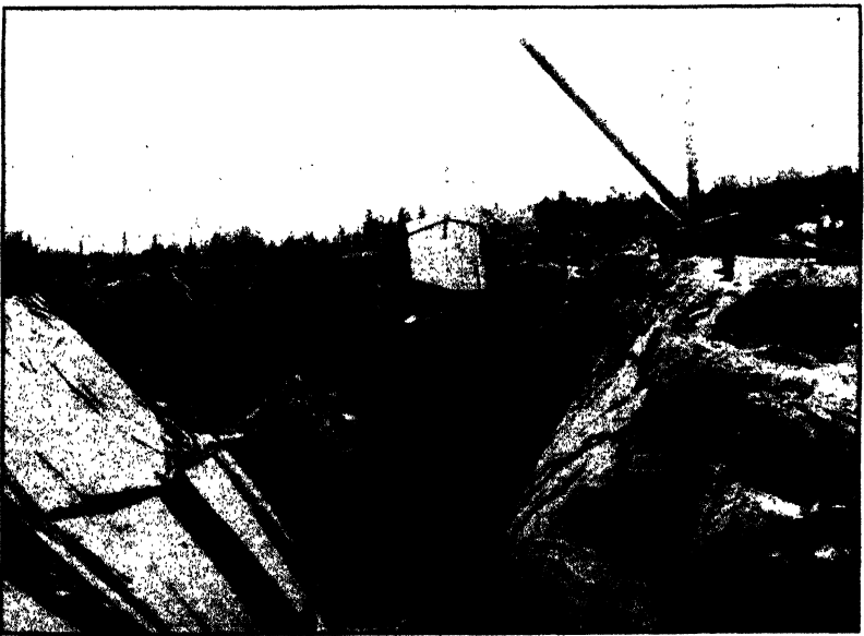
FIG. 2.—View in scythestone quarry, Pike Station, N. H. (Photo. lent by Pike Mfg. Co.)
